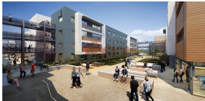
Orange Coast College's 800-bed project, constructed for $89 million.
