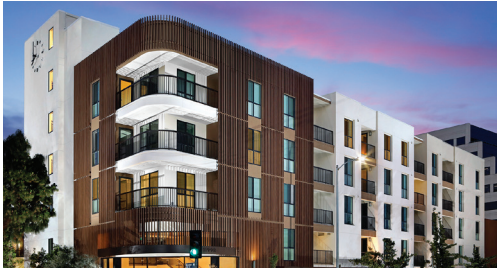
Missouri Place Thomas Safran & Associates City and County of Los Angeles
