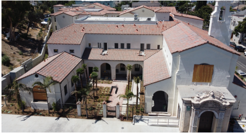
Washington View Apartments Western Pacific Housing, LLC City and County of Los Angeles
