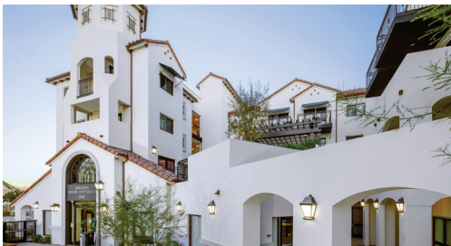
Arboleda Senior Apartments Meta Housing Corporation La Puente, Los Angeles County
